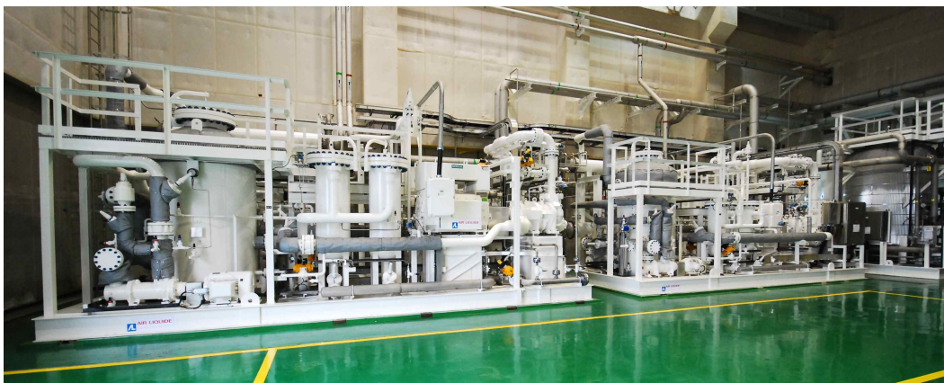
Fig. 1 Picture of the WCS in the helium plant room
