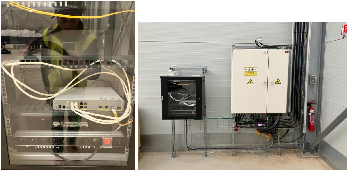
Figure 3 – Pictures of the existing B55.2 IT cabinet to connect cameras
