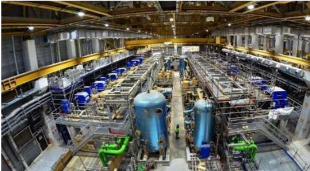
Cryoplant area / Warm Compressor Station
