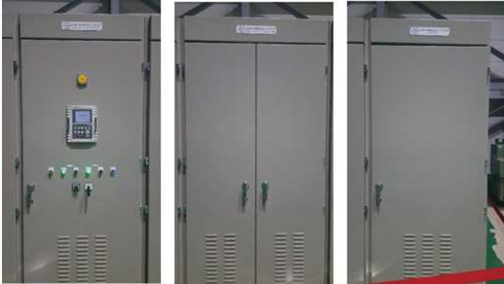
Pre-charge 저항, 필터 콘덴서&리액터, Damping resistor PNL
