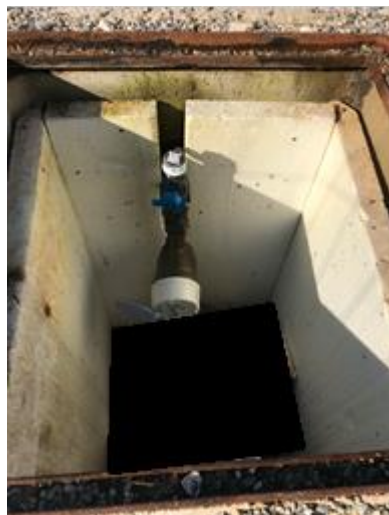
Figure 2: Potable water connection point in existing manhole
